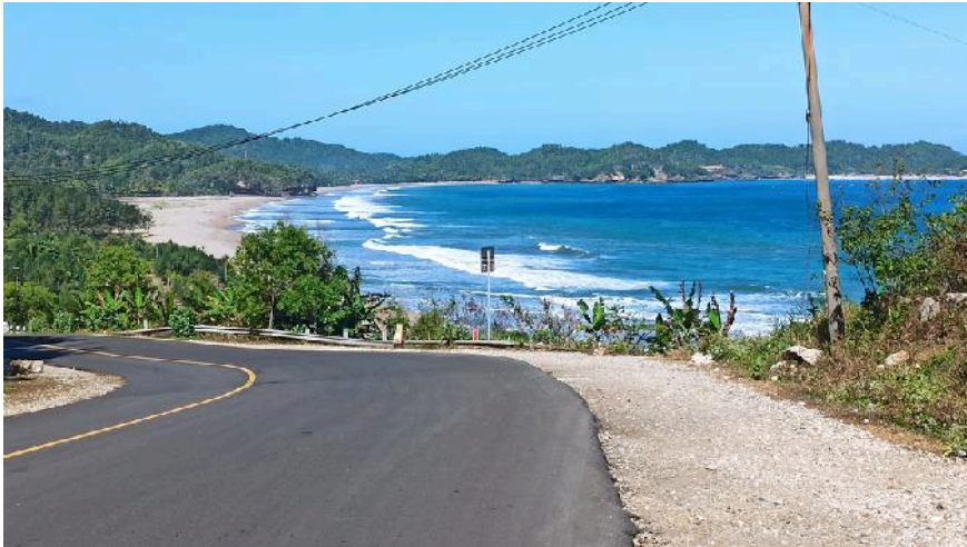
Figure 2.20 View From the Cliff Road (Source : Google Maps 2024)
