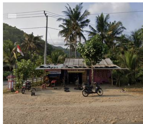
Figure 2.38 Motorcycle Repair Shop (Source : Google Maps 2024)
