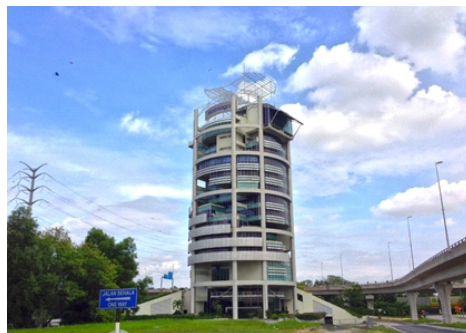
Gambar 2.33 Mesianaga Tower Sumber : Archdaily.com
