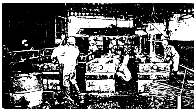
Gambar 5.9 Bekisting BJR
