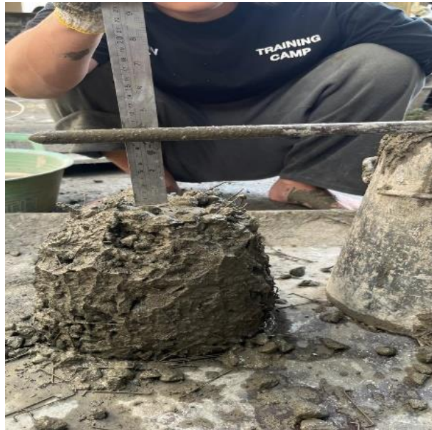
Gambar 5.11 Proses Pengujian Slump Beton
