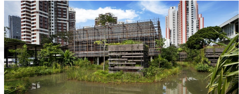
Gambar 2.37 Enabling Village, Singapore Sumber : Archdaily, 2016
