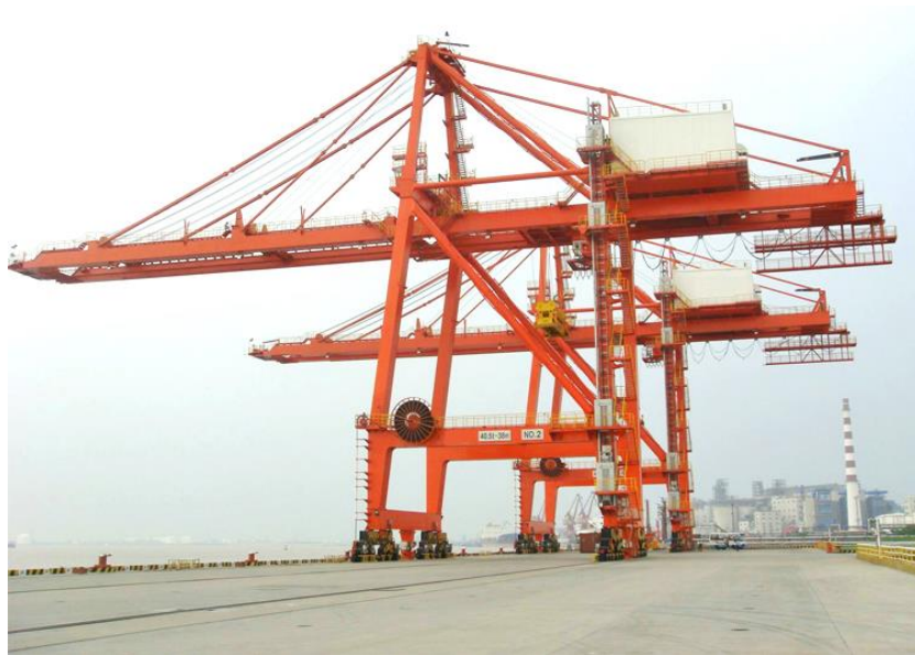
Gambar 3.2 Rail Mounted Crane
