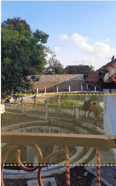
waste water treatment
