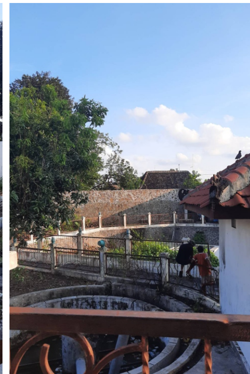
Abandoned space at west part of Plaza ngasem ( was formerly city waste water treatment) Source : Author,2021
