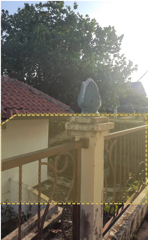
waste water treatment
