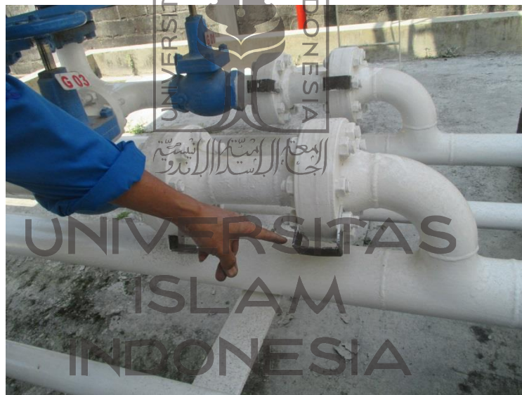
Gambar 5.18 sistem bonding area penimbunan
