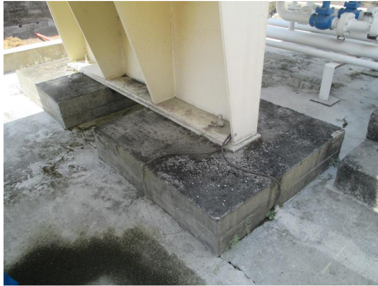
Gambar 5.17 sistem grounding area penimbunan
