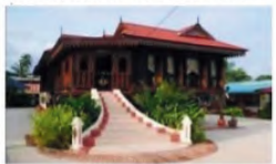
Fig 6.5 Staircase in Malacca house represents the social status and wealth of the house owner
