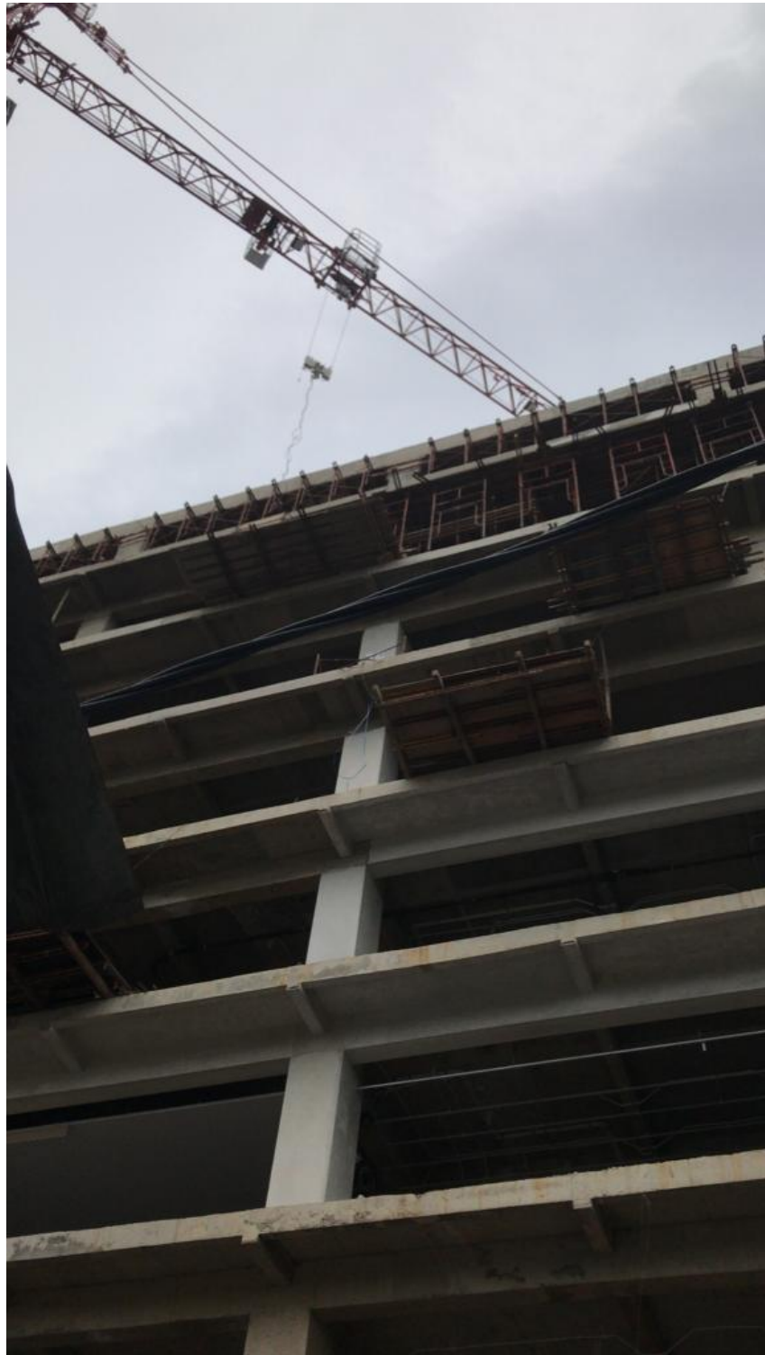
Gambar L-3.6 Proses Lifting Elemen Rangka Baja
