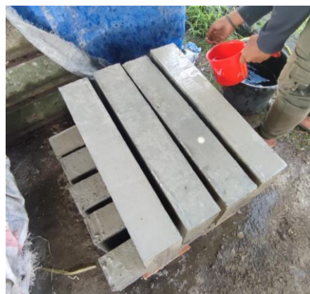
Gambar L 4. 12 Proses Curing Bata Ringan
