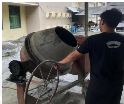
Gambar L.11.2 Proses Pencampuran ( Mixing ) Campuran Beton
