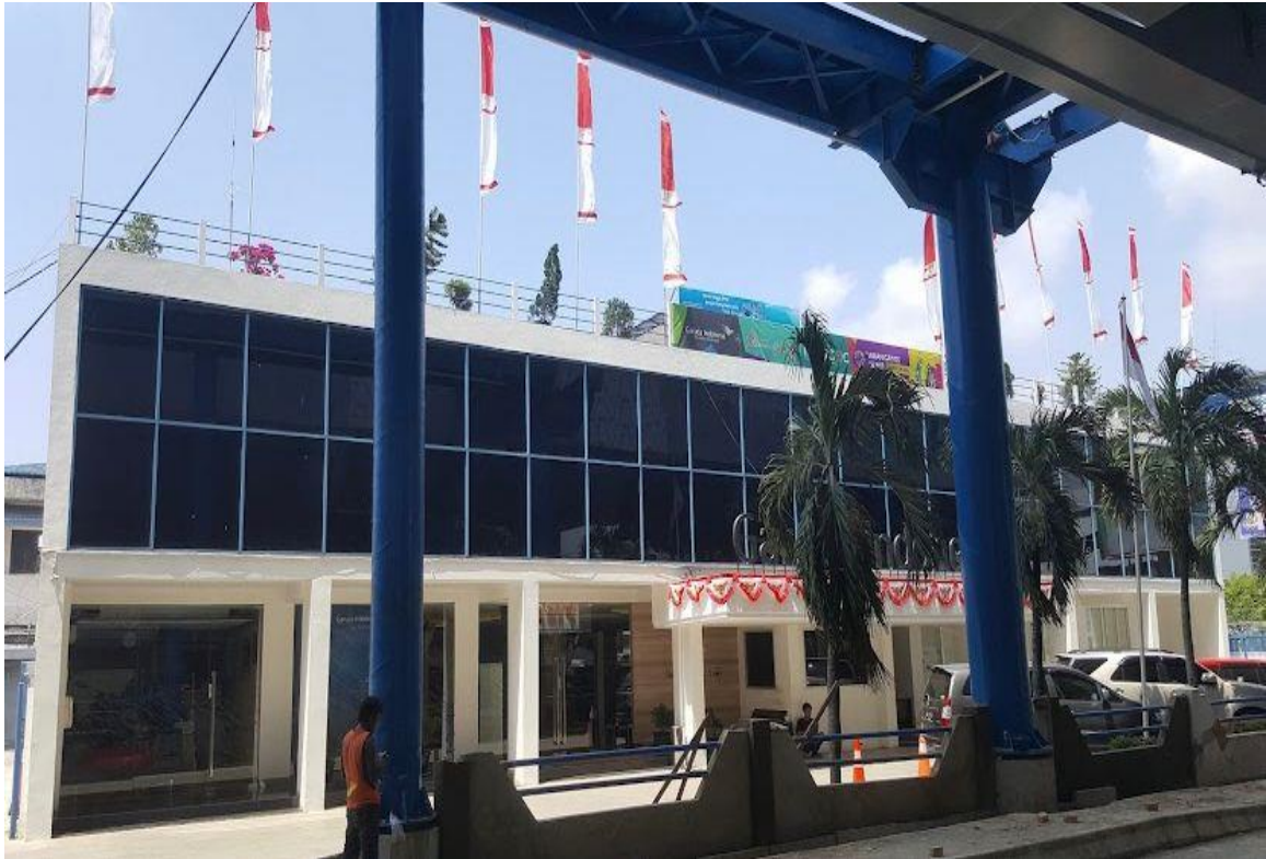
Gambar 2. Gedung PT. GIP
