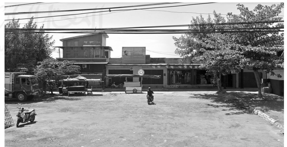
Figure 1.5. Conditions of retail kiosk Source : Google earth
