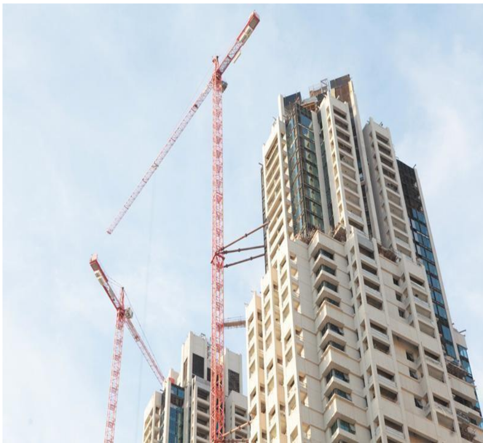
Gambar 3.4 Tied In Crane (Sumber: Construction week online.com )
