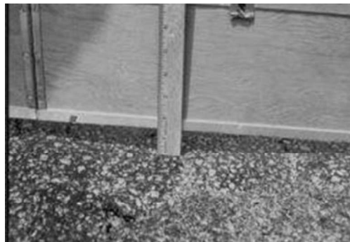
Gambar 3.28 Tingkat High Kerusakan Rutting (Sumber: Department of the Army, 1982 )
