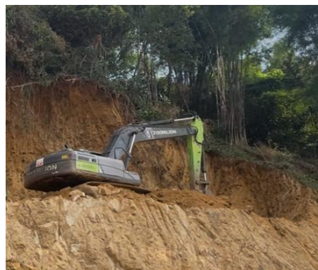
Figure 5. 7 Excavator Waiting for Dump Truck
