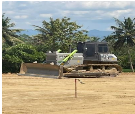
Figure 5. 9 Bulldozer waiting for material
