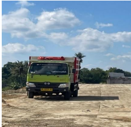
Figure 5. 8 Dump Truck Stops After Unloading
