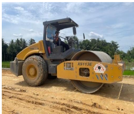
Figure 5. 11 Vibratory Roller on Break
