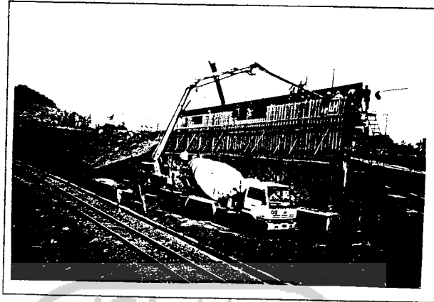
Gambar 5.3. Ready Mix Truck serta Concrete Pump
