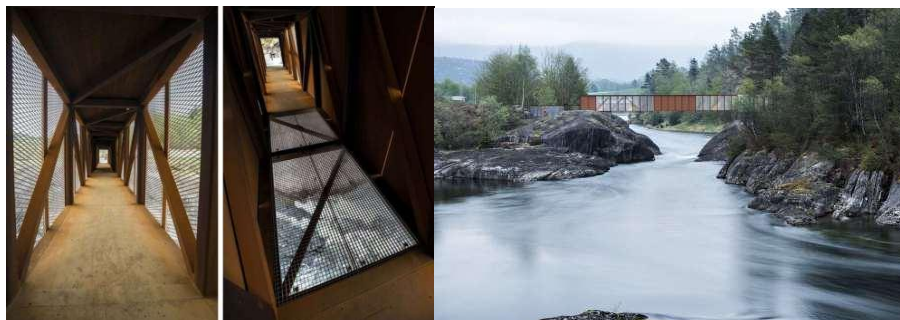
Gambar 17. Hose Brige Sumber : http://aasarchitecture.com/2014/06/hose-bridge-rintala-eggertsson-architects.html
