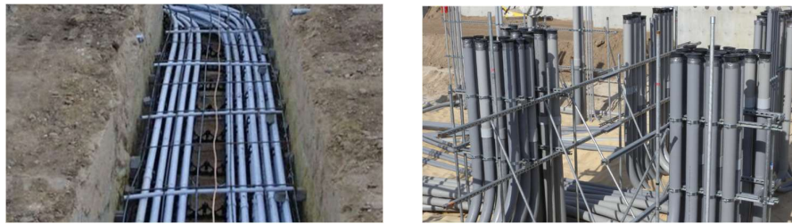
Gambar 3. 11 Conventional Position Frame ( Duct spacer )
