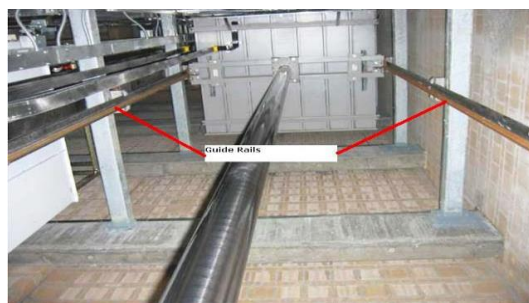
Figure 2.13 Guide Rails
