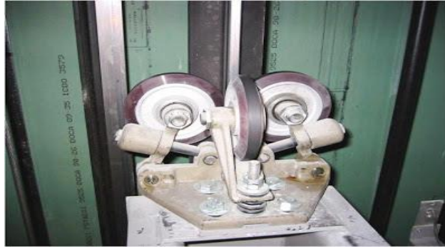
Figure 2.10 Roller Guides
