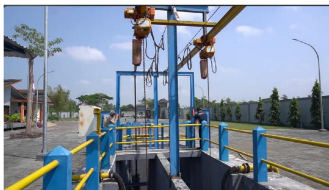
Gambar 2. 2 Aerated Grit Chamber
