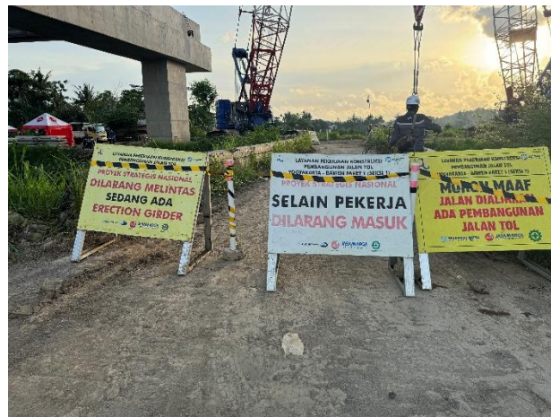
Figure 5. 3 Provision of Signs in Specific Areas (Source: Personal Documentation)
