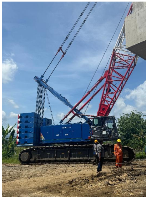
Figure 3. 3 Crawler Crane (Sources: Personal Documentation)
