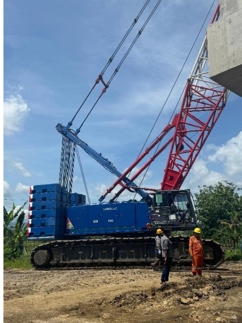
Figure 5. 5 Track Crane Inspection (Source: Personal Documentation)
