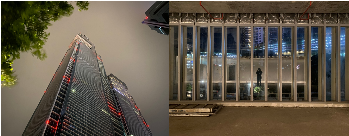
Figure 2.1.2 Autograph Tower Survey Source : Author, 2025
