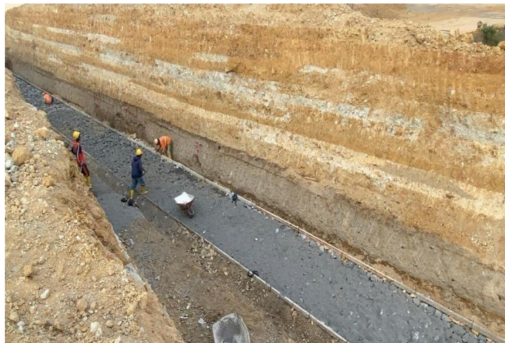
Gambar 3. 6 Proses Blinding Stone
