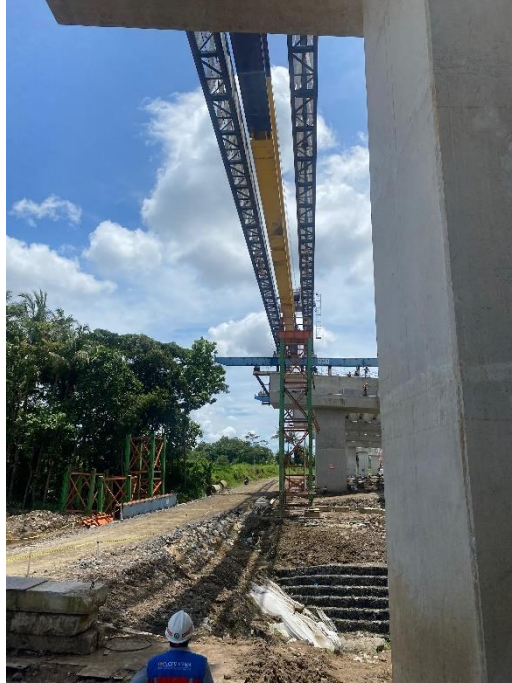
Gambar L-9.5 Proses Lifting Erectiong Girder
