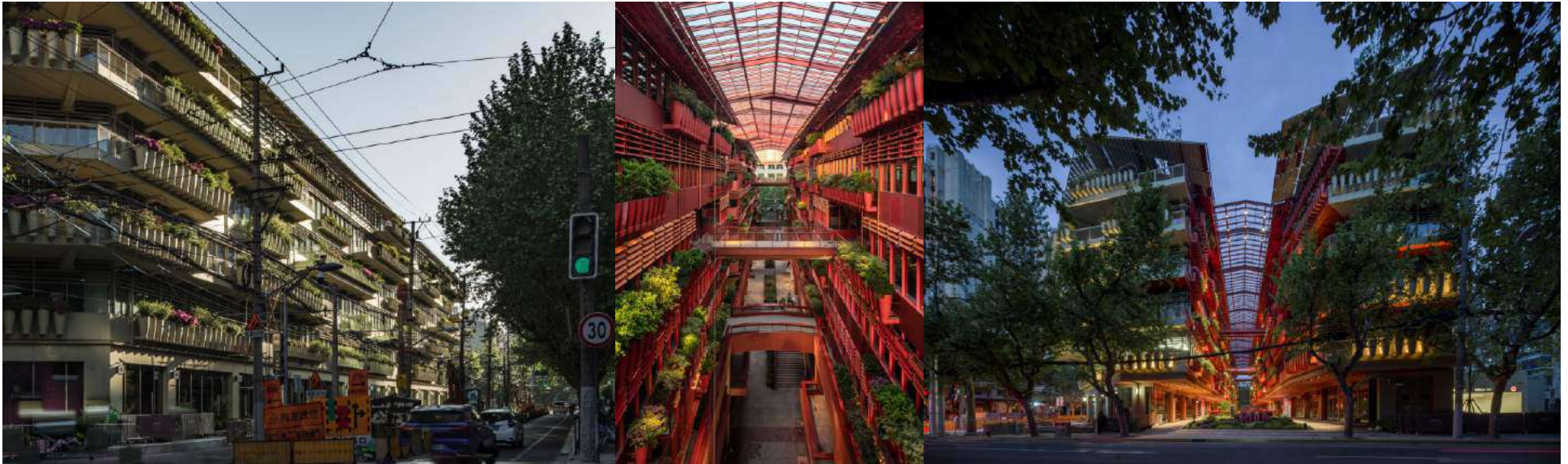
Gambar 17 Eksterior Henderson Cifi Tiandi Sumber : https://www.archdaily.com/961565/henderson-cifi-tiandi-ateliers-jean-nouvel?ad_medium=gallery
