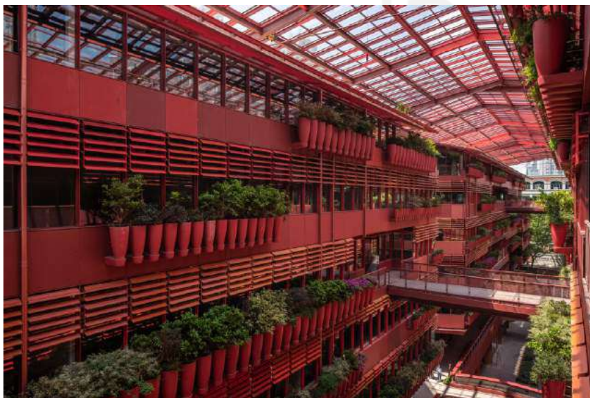
Gambar 18 Interior Henderson Cifi Tiandi Sumber : https://www.archdaily.com/961565/henderson-cifi-tiandi-ateliers-jean-nouvel?ad_medium=gallery
