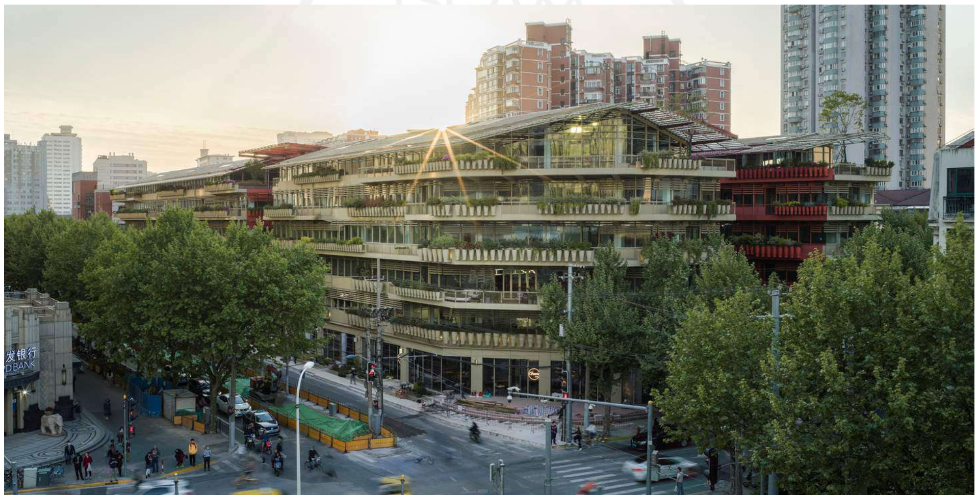
Gambar 19 View Luar Henderson Cifi Tiandi Sumber : https://www.archdaily.com/961565/henderson-cifi-tiandi-ateliers-jean-nouvel?ad_medium=gallery
