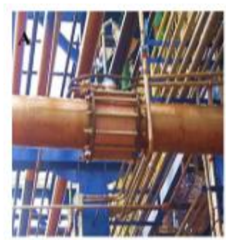
Gambar 5. 2 Automatic flow rate meter at the outlet
