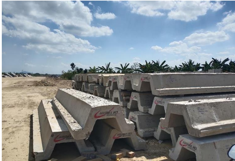
Gambar 3.3 Corrugated Concrete Sheets Pile (CCSP)
