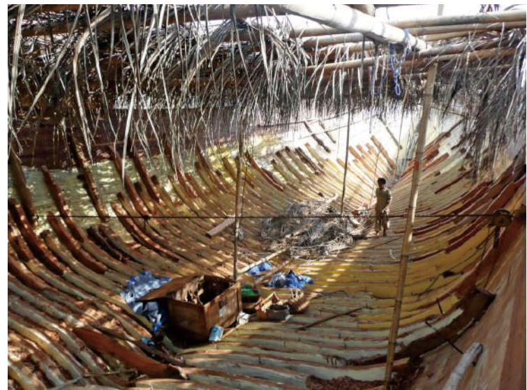
Picture 2.15 Pinisi Construction Process Source: Author
