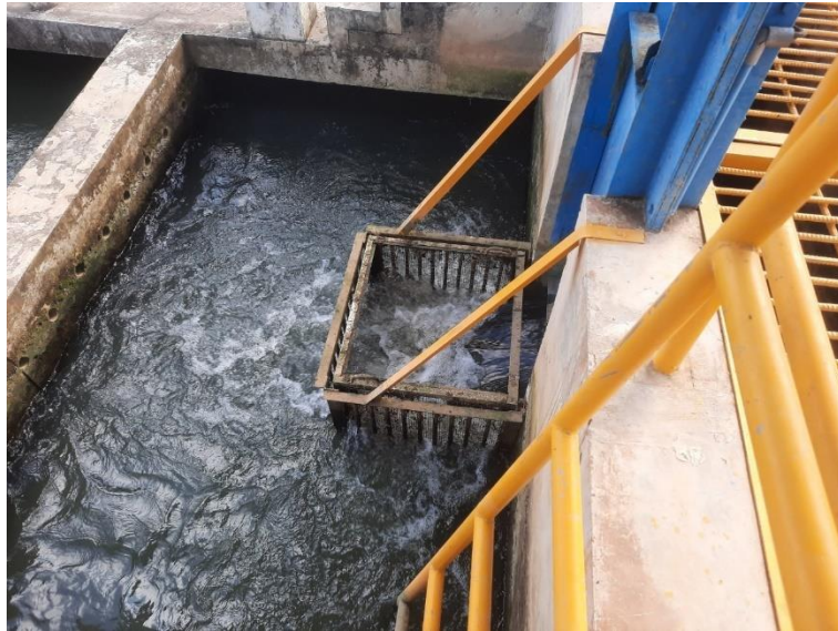
Gambar 4. 8 Inlet Unit Bak Prasedimentasi
