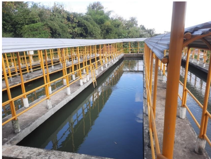
Gambar 4. 9 Bak Unit Prasedimentasi
