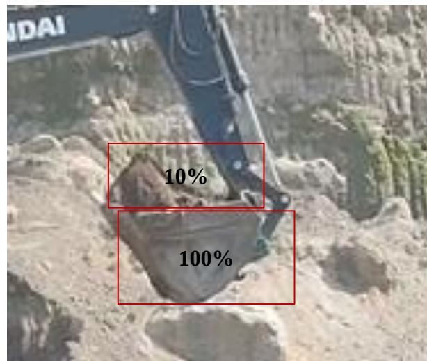
Gambar 5. 3 Bucket Excavator Hyundai Terisi 110%
