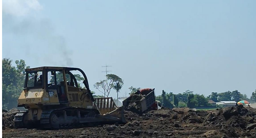
Lampiran 45 Bulldozer Meratakan Tanah Hasil Bongkaran Dump Truck
