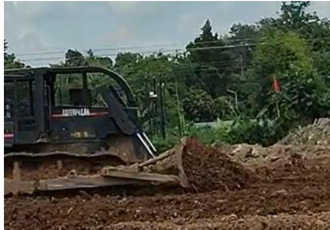
Gambar 5.5 Blade Bulldozer Terisi 100%
