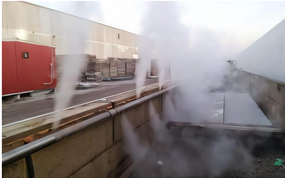
Gambar 3.3 Metode perawatan steam curing beton (Sumber: Internet)
