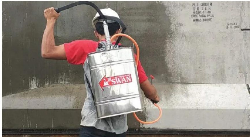
Gambar 3.6 Metode perawatan curing compound beton (Sumber: Internet)
