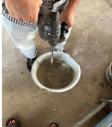
Gambar 4. 18 Pencampuran Material Kedalam Foaming Agent
